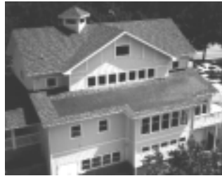
Building integrated photovoltaics. Photo courtesy of John Haigwood.
